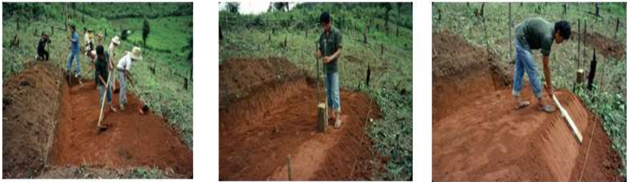
Figure 10 Compaction of fill soil
