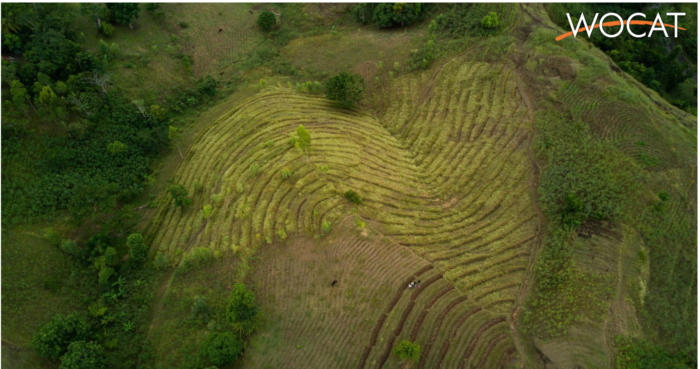
Slope stabilisation and progressive terracing with vetiver grass (Joana Eichenberger)
